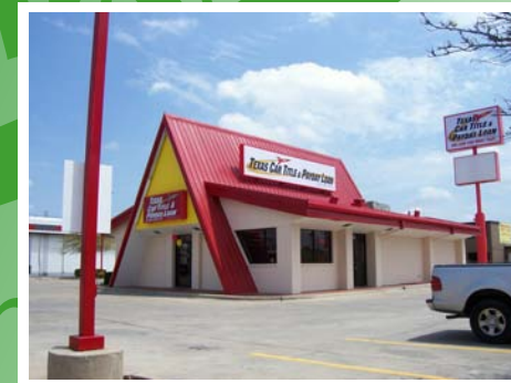
Pole Sign & Cabinet Signs
